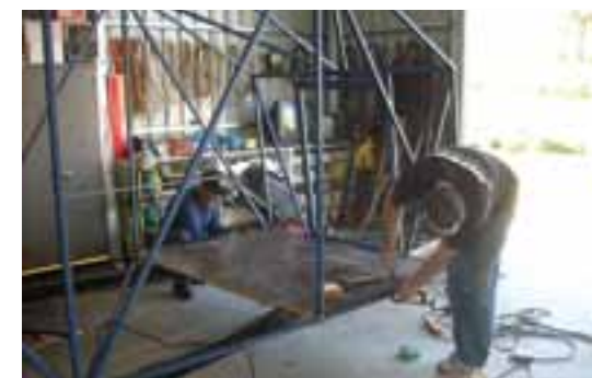
Installing the plywood floor.
